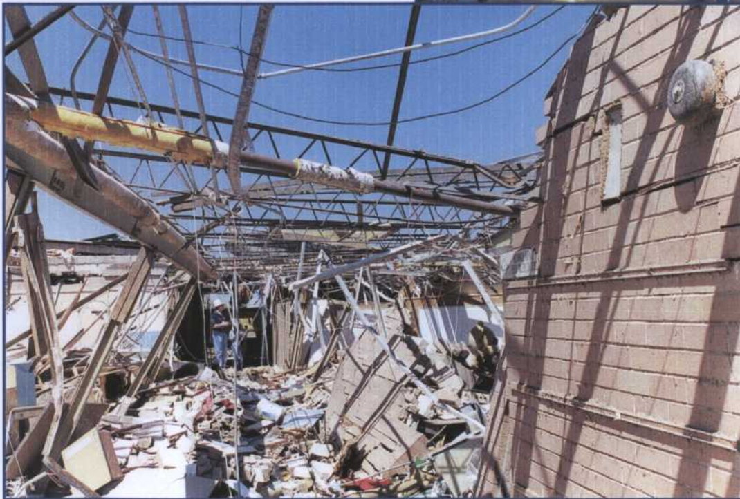
Figure 6-35. Kelly Elementary School, Moore, Oklahoma, place of refuge – corridor with clerestory windows. These interior corridor walls had brick masonry up to a height of approximately 7 feet. Glass extended from the top of the brick masonry to the top of the wall.
