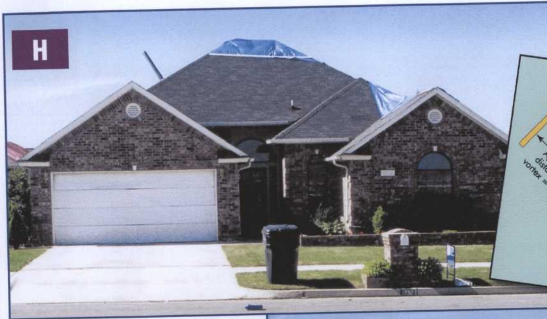
Figure 4-22. Home in Moore, Oklahoma, with partial roof loss and garage door in place (H) vs. home with total roof loss due to garage door failure under positive pressure (A).
