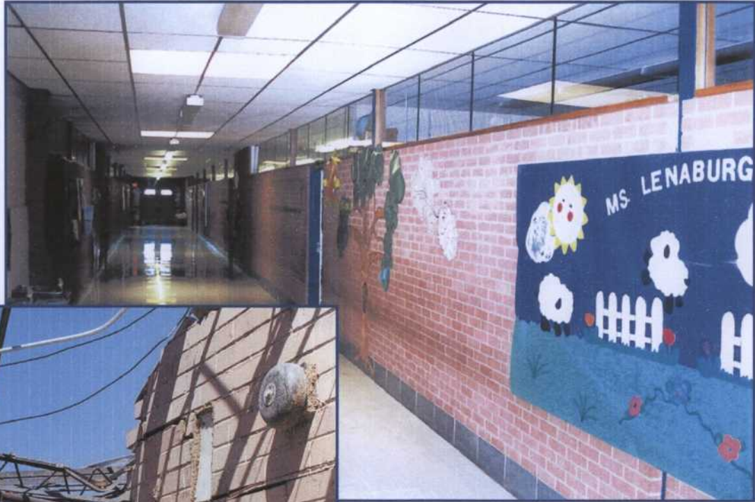
Figure 6-34. Northmoor Elementary School, Moore, Oklahoma, place of refuge – corridor with clerestory windows. This corridor offers little protection from tornadoes as shown in a school of similar design in Figure 6-35.
