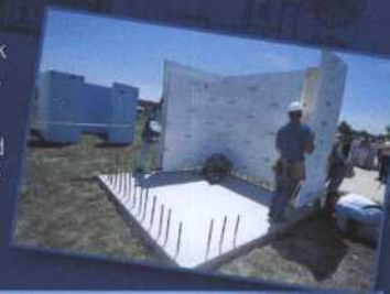
Workers lift insulating concrete form (ICF) section into place over concrete slab foundation.
