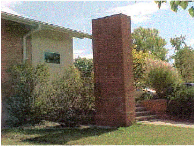
Figure 2. The two sides of the brick structure to which the metal facing would be applied. Facing Southeast.
