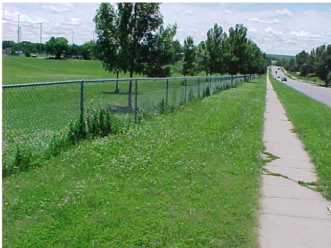
Fence line at Holcom Park – Needs to be sprayed with Round-up to eliminate weeds in fence
