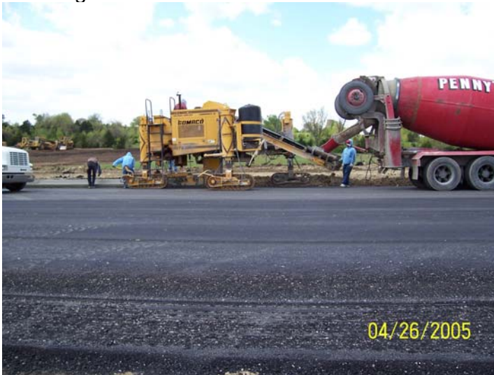
Curb & gutter construction
