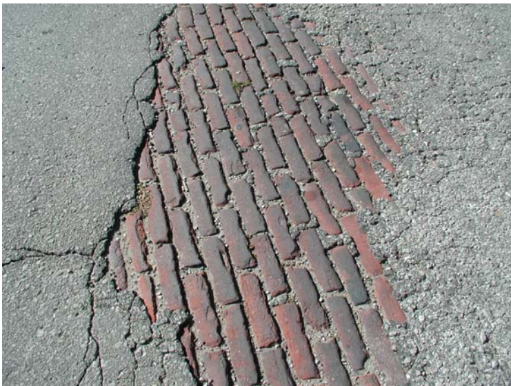
Existing street has asphalt overlaid on top of the bricks which will be removed and re-laid.
