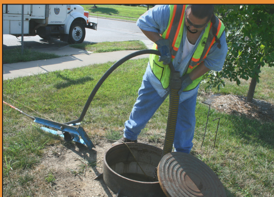
Technician removes lid to clean West Lawrence sewer line with high-tech forced water equipment.
