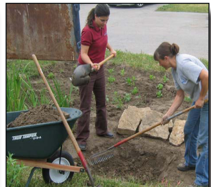
City employees built a rain garden at a city facility.
