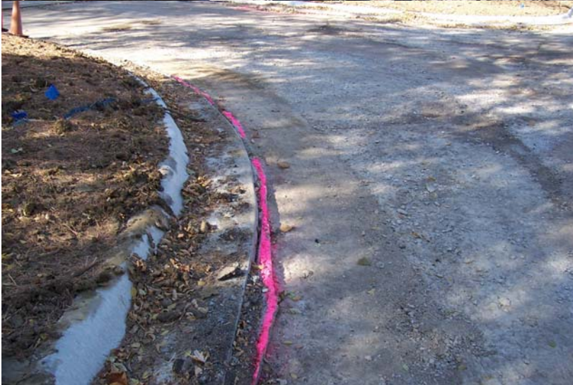
Area marked in pink is excess concrete ("slobbers") that prevent adequate depth of overlay at the edge of the pavement.
