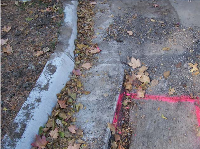
Back of curb and front edge of gutter do not align on each side of joint.
