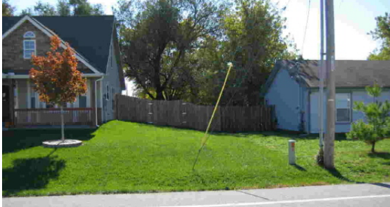
Another—where does this house drain? Onto the older neighbor, of course. Strange as this may seem, the City of Lawrence building codes not only allow but encourage this practice.
