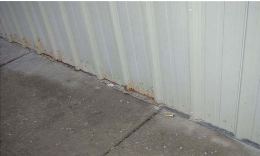
South Elevation Wall Rust
