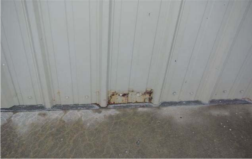
South Elevation Wall Rust
