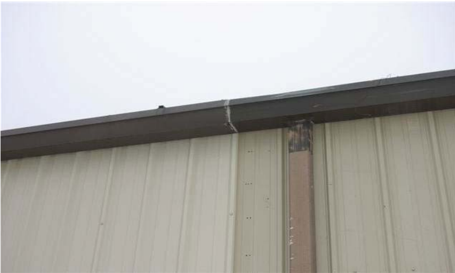
Gutter Leaks
