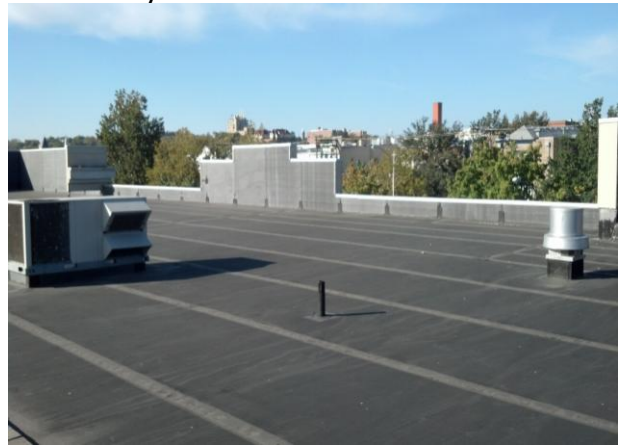
Maintenance to Community Health Building Roof
