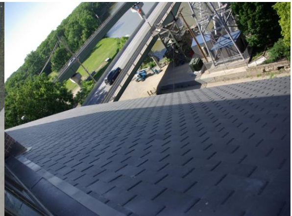
City Hall Roof replacement
