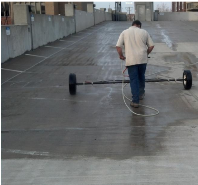
Sealing concrete NH parking garage
