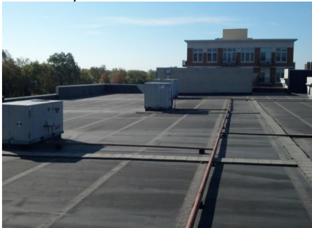
Maintenance to Community Health Building Roof
