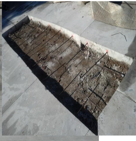
Full depth repair RF parking garage
