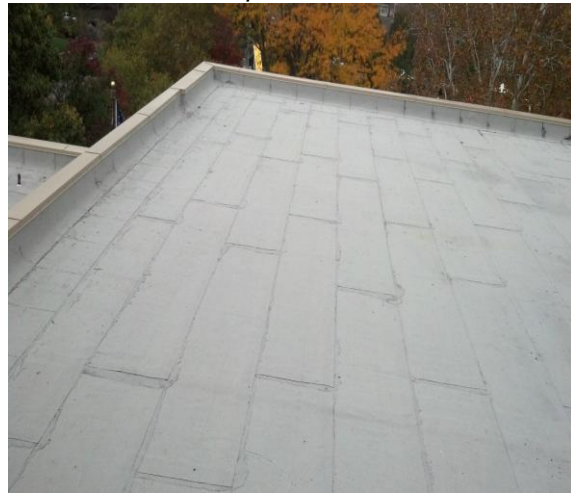
Senior Center Roof
