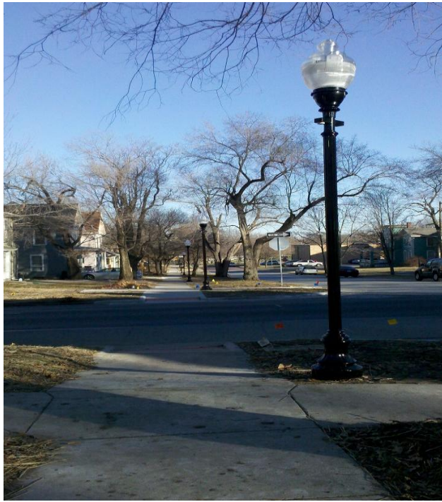
12th Street Lighted Pathway
