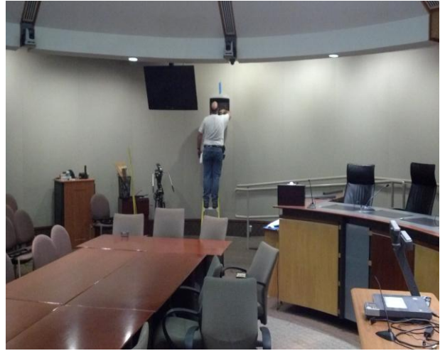
City Commission room remodel
