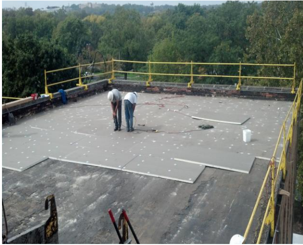
Senior Center roof
