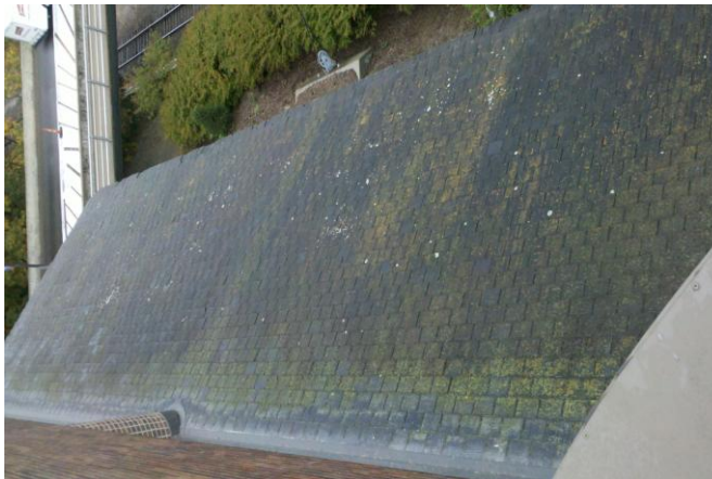
City Hall Roof replacement
