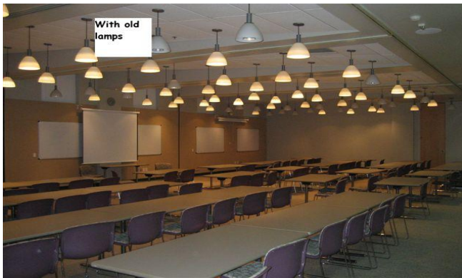
Health Building original lighting
