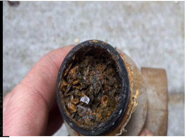
Replaced Fire Sprinkler lines at New Hampshire Parking Structure
