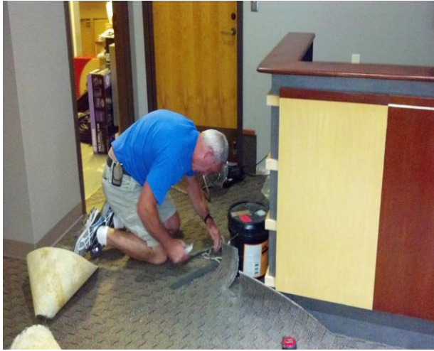
City Commission room remodel
