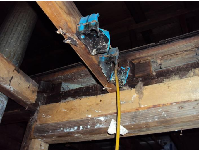
Fire damaged electrical boxes in ceiling (1 st floor)
