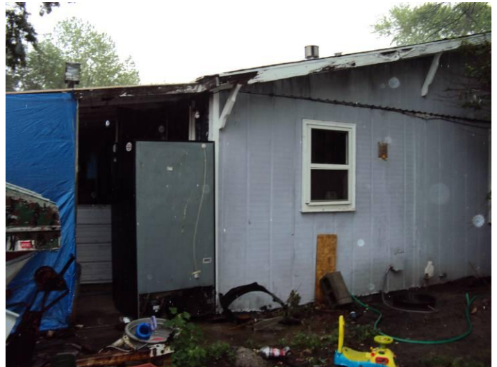
Refrigerator – plugged in and exposed to weather
