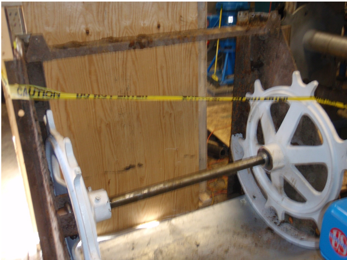
Boot section with new lower chain sprockets and bushings installed
