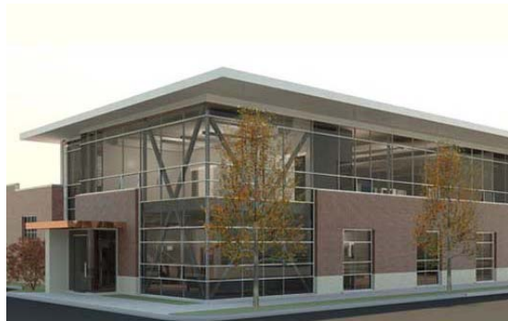
1040 Vermont Street office
