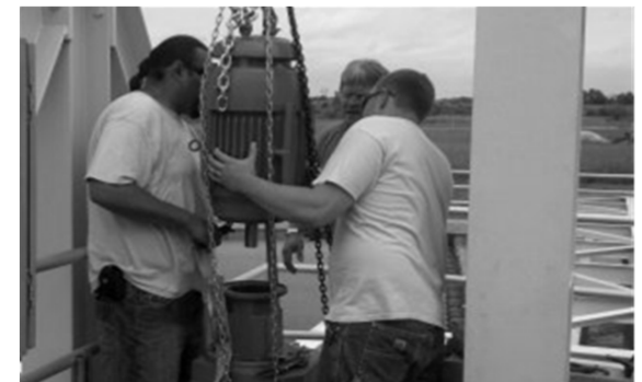
CLINTON WATER TREATMENT PLANT
