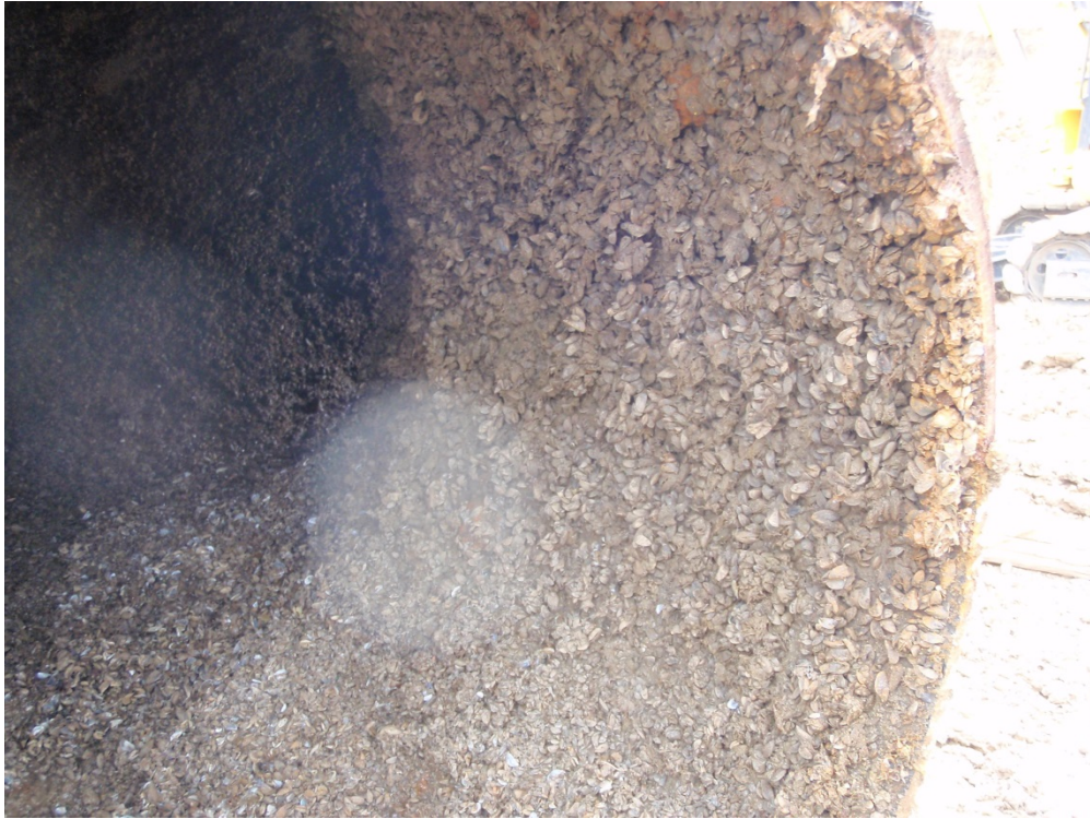
March 2016 - Zebra Mussel Accumulation Inside 36" Diameter Raw Water Transmission Main
