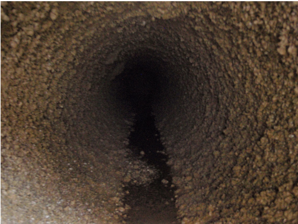
March 2016 - Zebra Mussel Accumulation Inside 36" Diameter Raw Water Transmission Main
