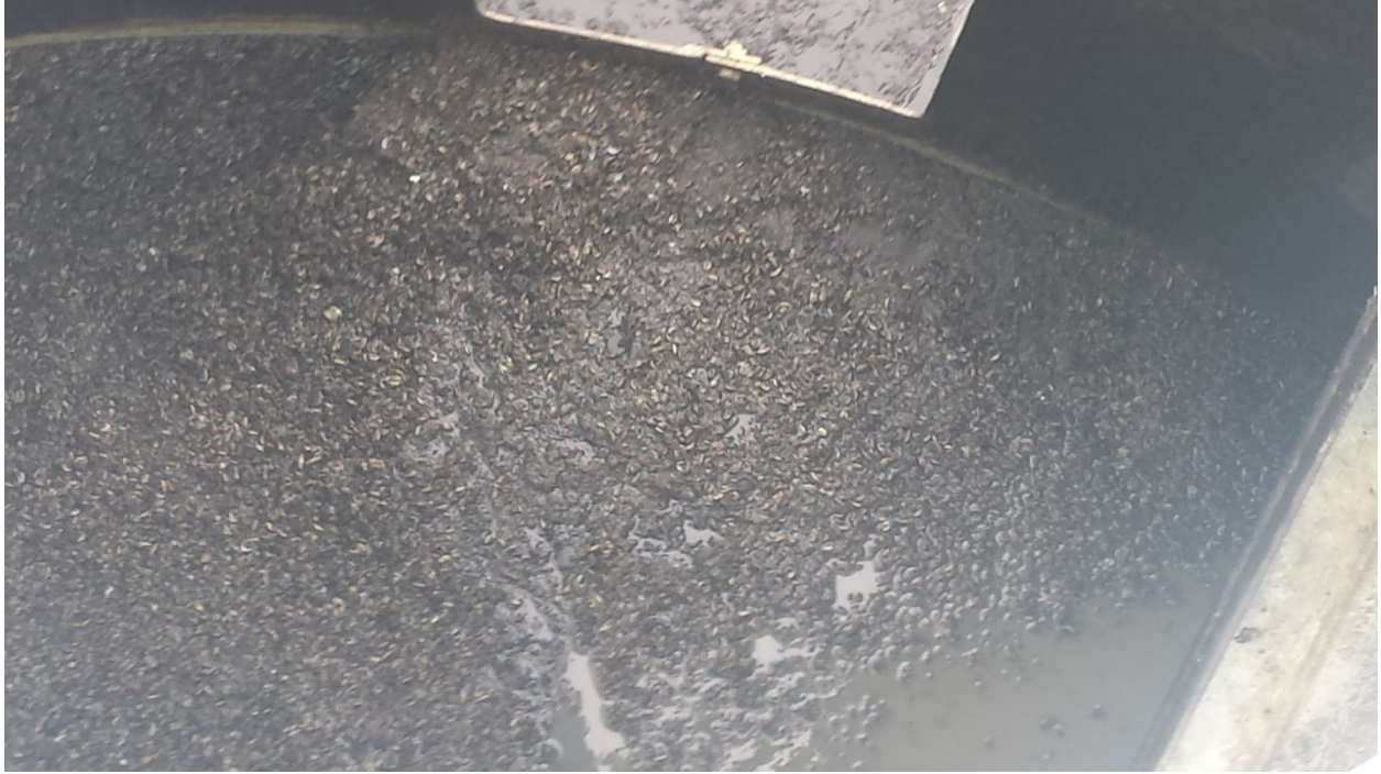
March 2016 - Zebra Mussel Shells Found in Clinton Water Treatment Plant Process Equipment
