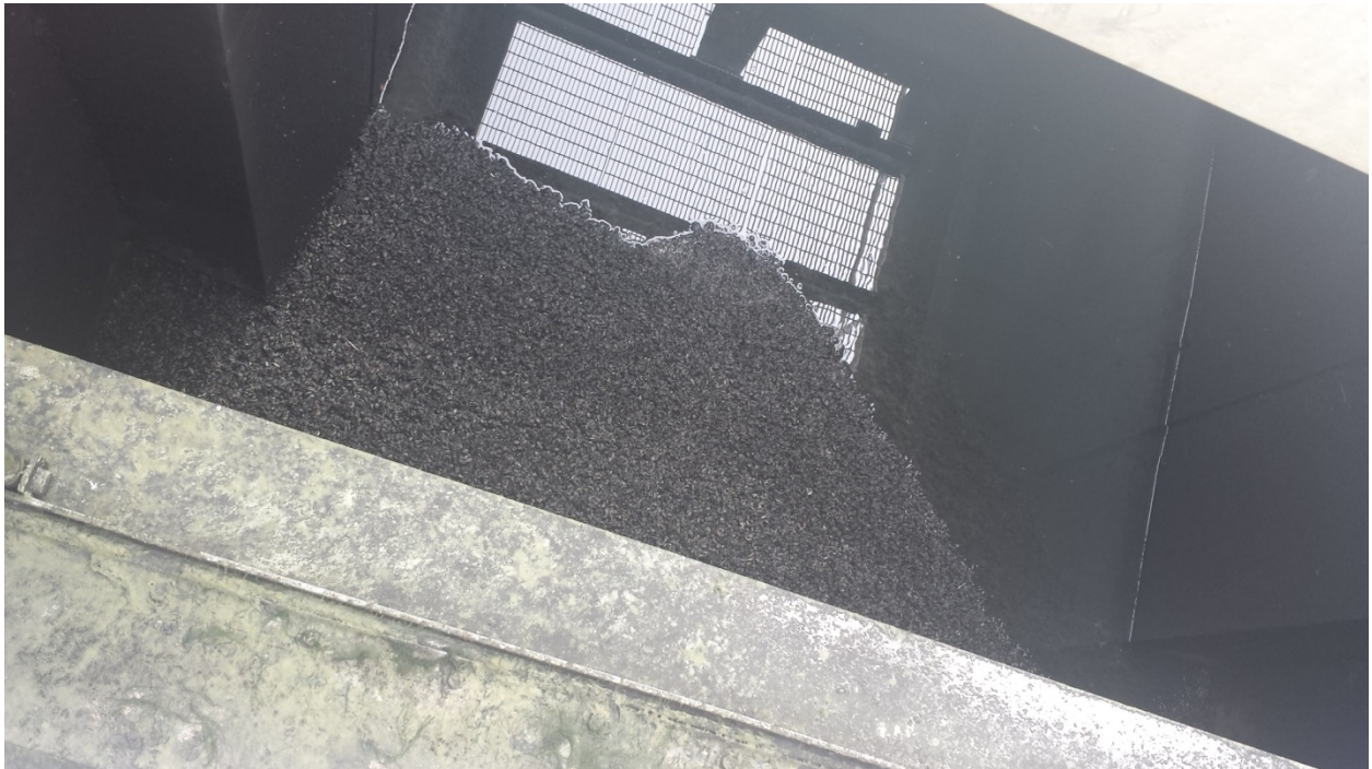
March 2016 - Zebra Mussel Shells Found in Clinton Water Treatment Plant Process Equipment
