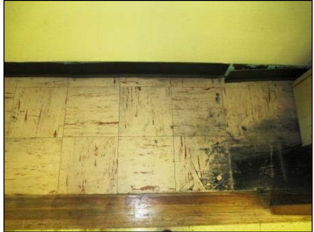
Freight office closet 9x9 floor tiles/mastic
