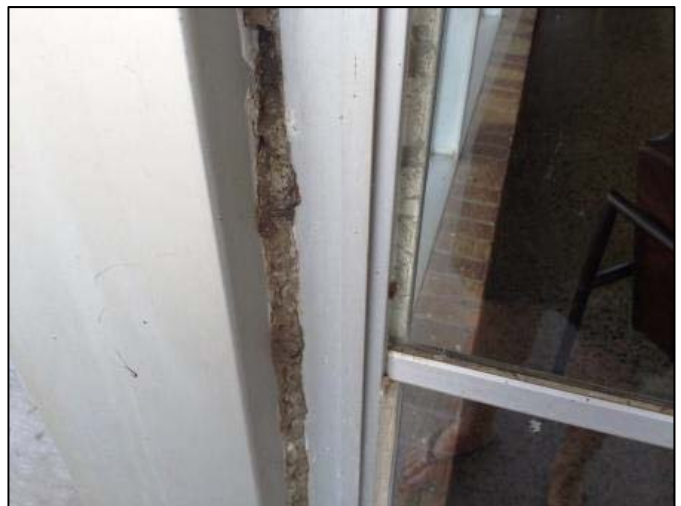
Caulk at exterior window
