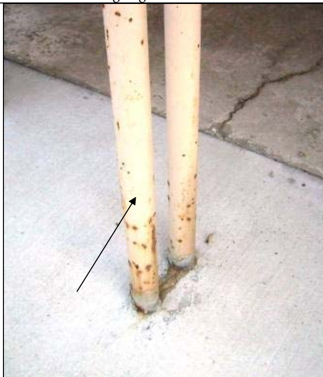
Deteriorated LBP on the exterior columns
