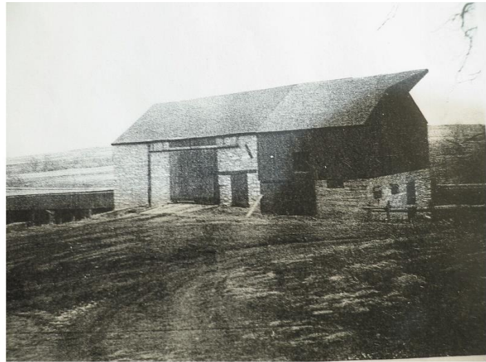
Grover Barn-south side-with addition on right (east) date unknown
