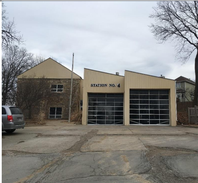
Grover Barn is on the Left of the Photo and the Fire Station Addition is on the Right, 2018
