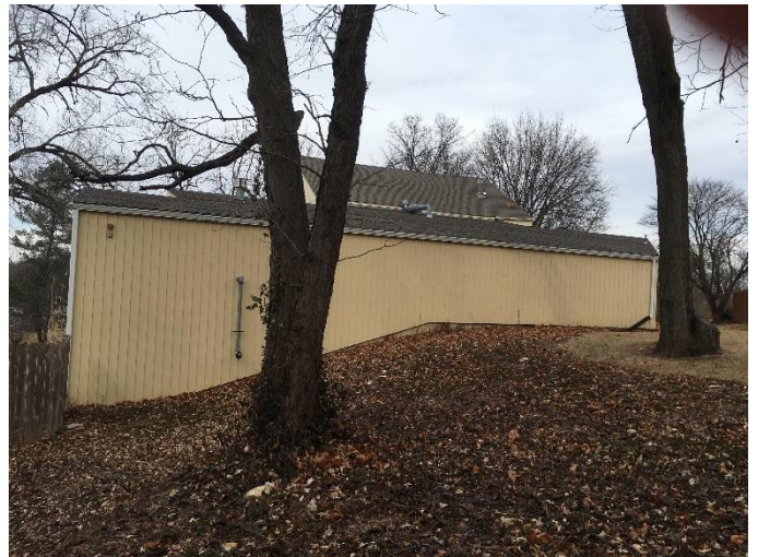
Embankment to the South of the Fire Station Addition 2018
