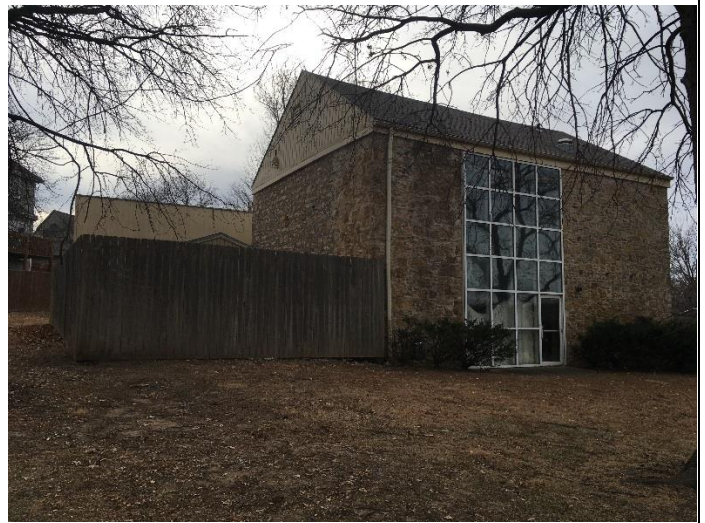
Northeast Elevation of Grover Barn, 2018
