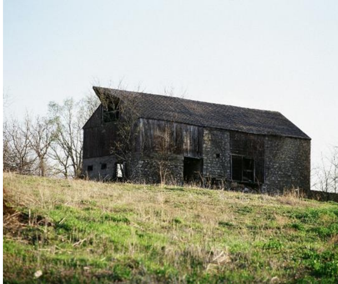
Northeast Elevation of Grover Barn, 1981 (Photo by Clay Kappelman)
