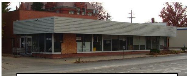
1040 Vermont Street Before Renovation
