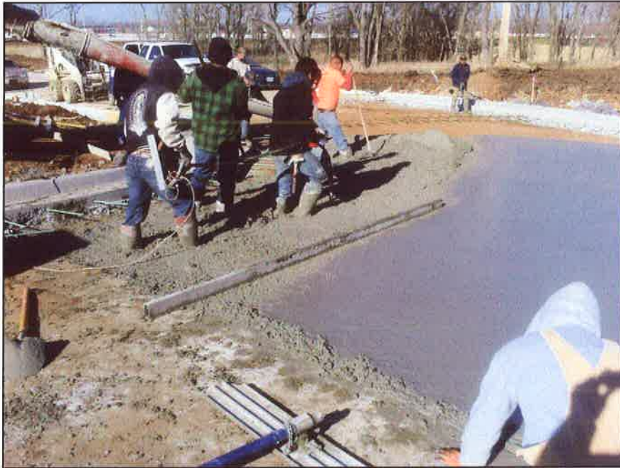
Vibrating concrete.
