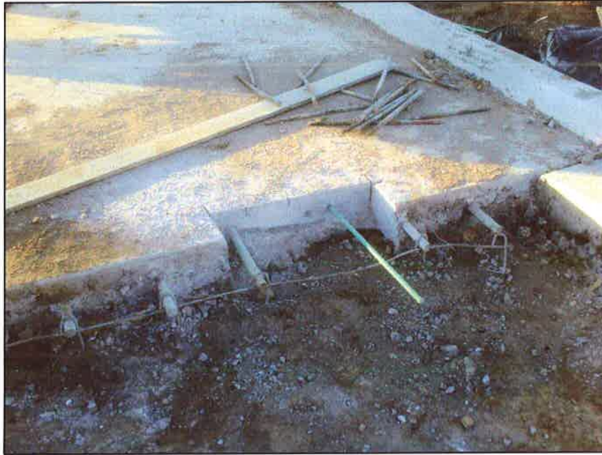
Construction joint on George Williams Way.
