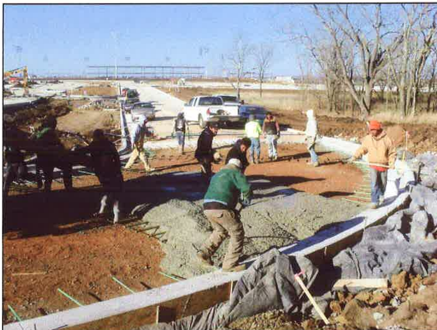
Placing concrete.
