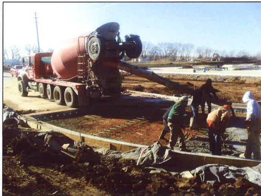
Began placing 10" concrete pavement.
