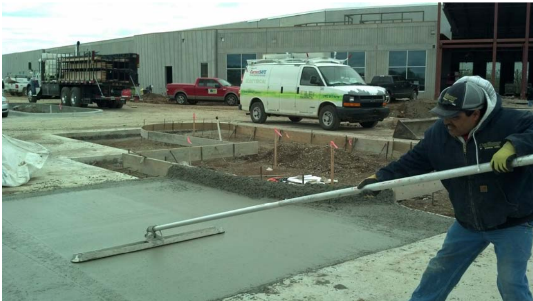
Parking and curb pour for parking in front of Rec Center
