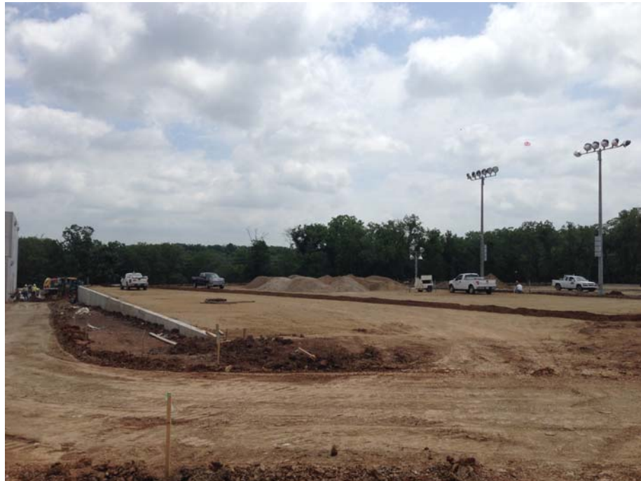
Beginning of tennis court construction
