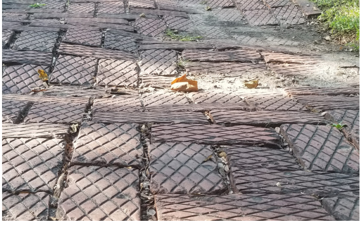
Non-Level Brick Cross Slope
