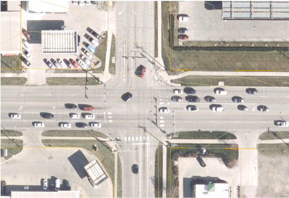
Figure 34: Overhead View of E 23rd St & Haskell
