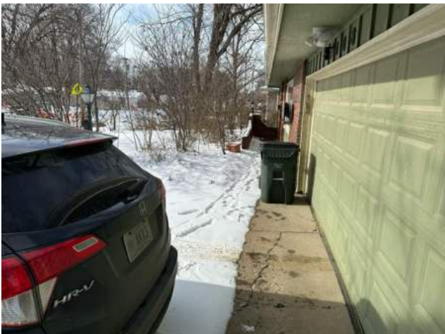
Exterior Side A Garage & Walkway
