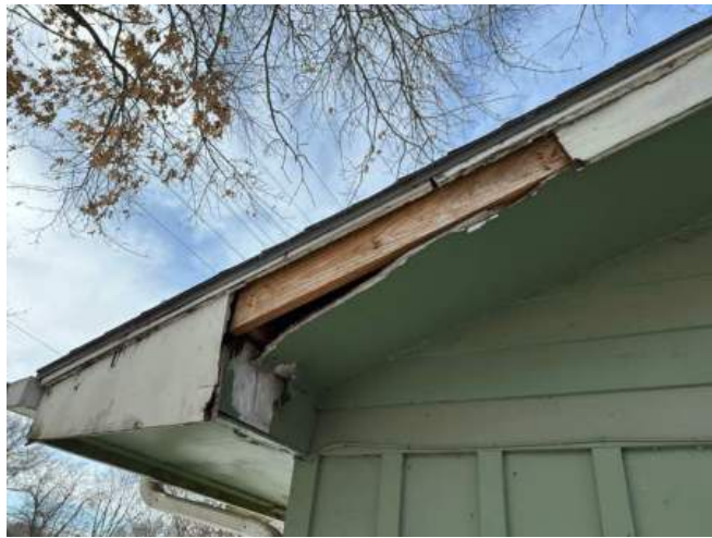
Exterior Side D Soffit & Fascia 2
