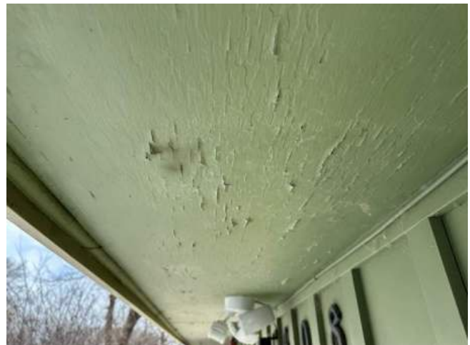
Exterior Side A Soffit
