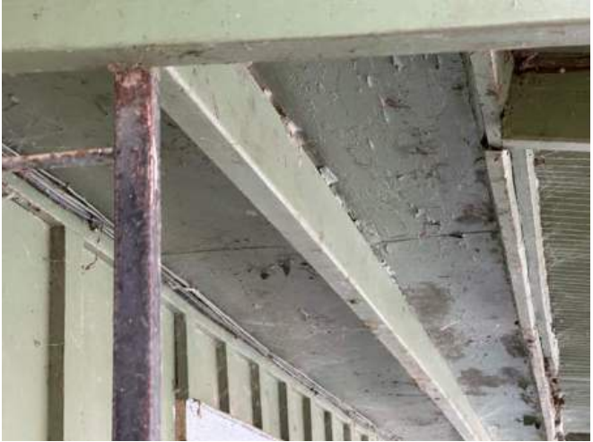
Exterior Side C Soffit & Fascia
