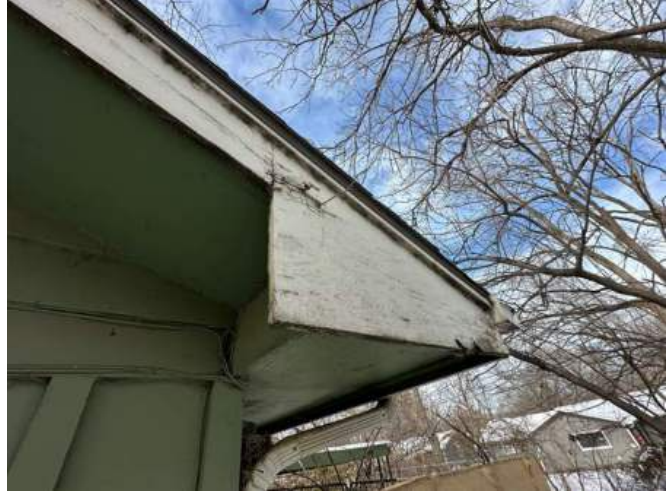
Exterior Side D Soffit & Fascia 1
