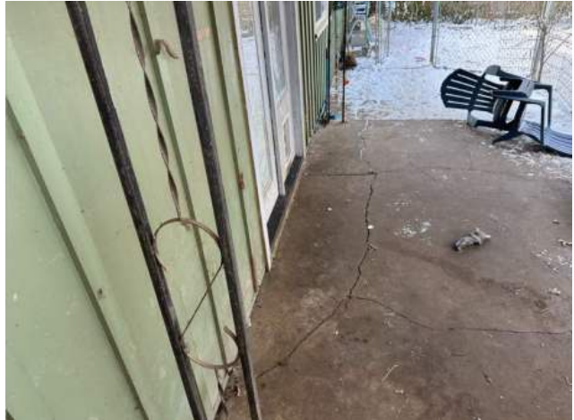
Exterior Side C Porch & Walkway
