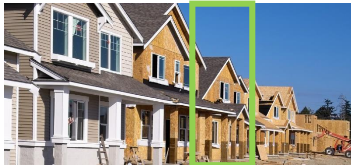
Fig. 20-9-C. Example of New Construction of a LERU or Affordable Unit In a Market-Rate Development
