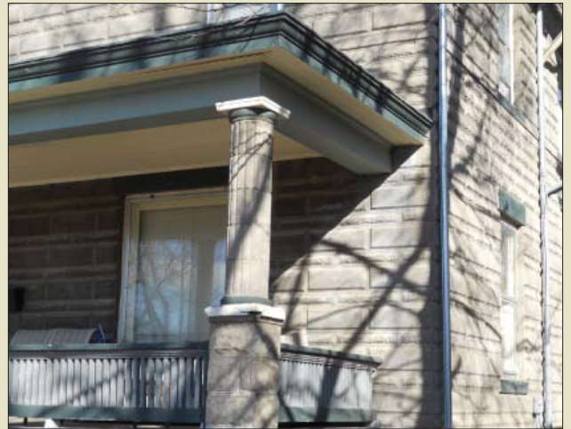
The load being supported by the columns should be expressed in the design of the structure. Columns and their bases should be evident.
