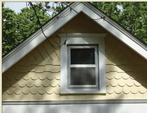
Wood shingles used on gable end.
