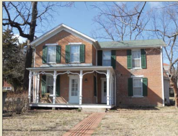
Brick is a common wall material.
