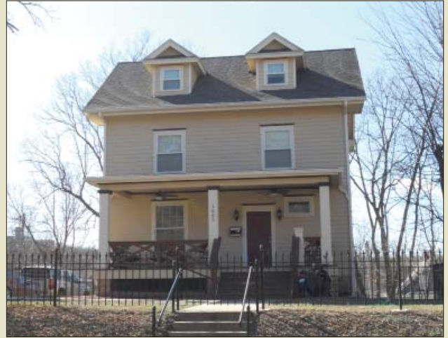
Dormers should be appropriately scaled so not to overwhelm or dramatically change the character.
