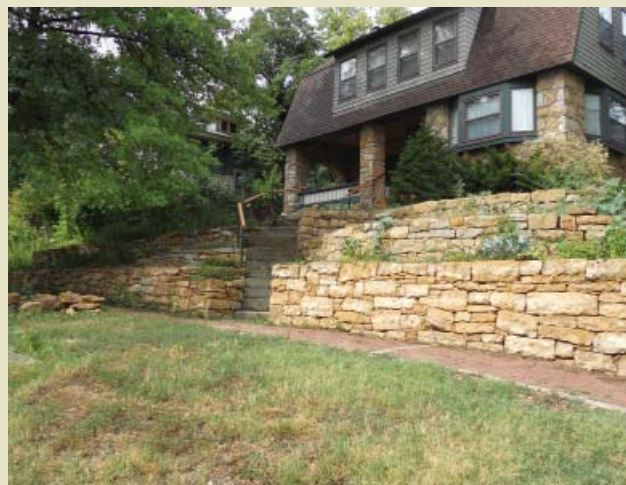
A good example of a stepped retaining wall in Oread.
