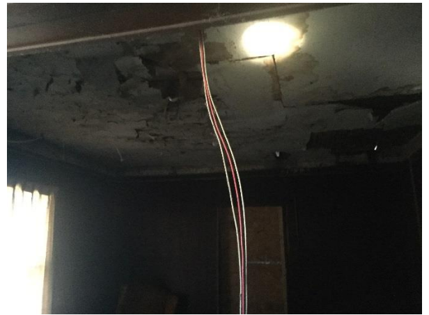
SW room, ceiling damage/partial collapse, hanging electrical wiring
