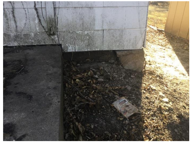
West elevation, foundation breaks/cracks
