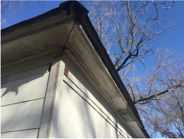
SW corner of structure, rotting roof materials
