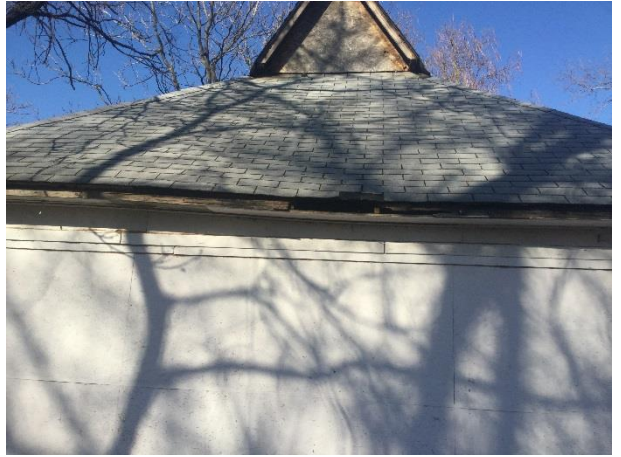
South side of structure, rotting roof materials
