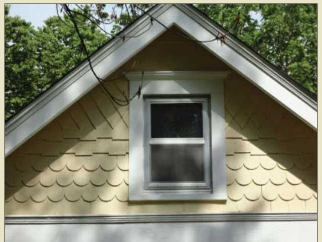
Wood shingles used on gable end.
