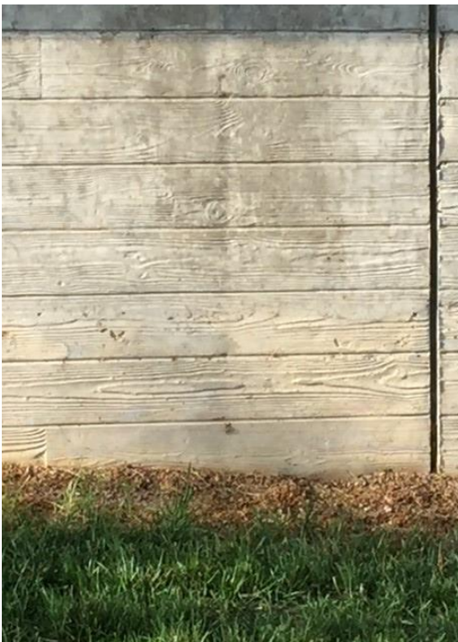
Details of the Board Formed Concrete on the Library Building
