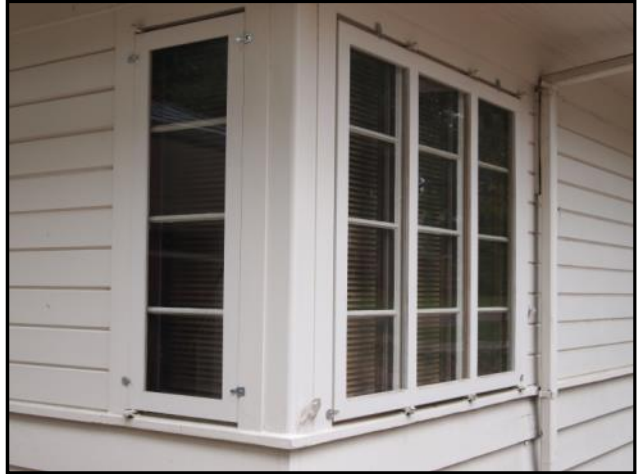
Casement windows like these are found throughout the house. The current owners added the storm windows. (Photo by L. Crick)
