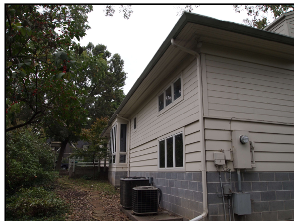
Rear Addition showing the CMU foundation wall and the similar siding treatment (Photo by L. Crick)
