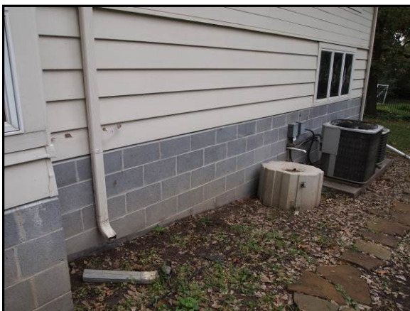
Rear Addition showing the CMU foundation wall and the similar siding treatment (Photo by L. Crick)
