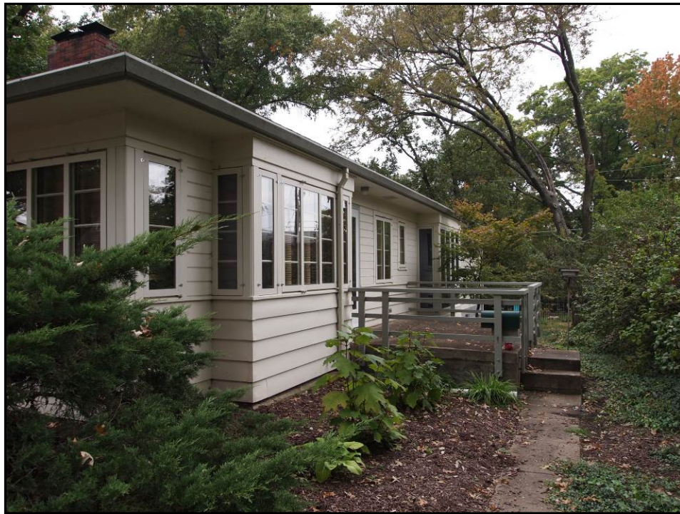
East elevation – the addition mimicked the protruding bay of the original house, but altered its window pattern (Photo by L. Crick)
