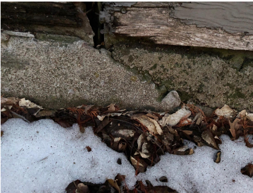
CRACKED FOUNDATION ON EXISTING GARAGE
