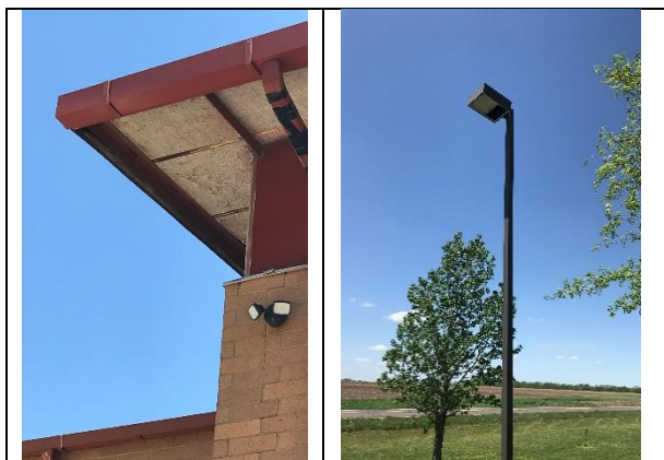
Figure 6. Exterior lighting; wall mounted security lighting on the left, driveway lighting on the right.
